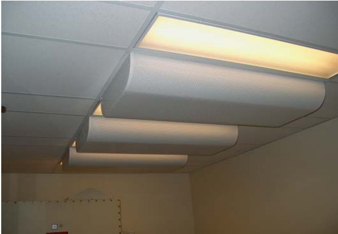
An example of the low velocity radial diffuser
